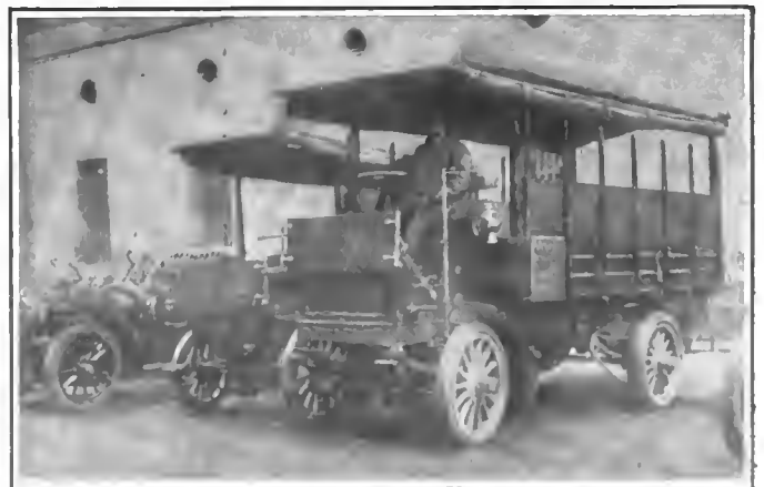
KNOX AIR-COOLED GASOLINE 16-20-H.P. TRUCK.
